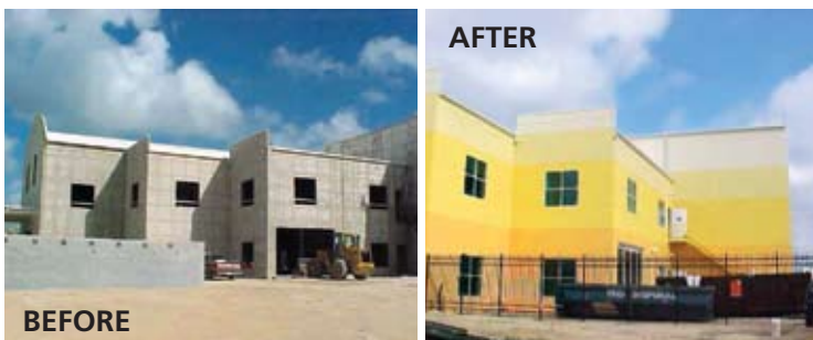
Tilt-up commercial project using 657 - StoCoat™ Acryl Medium as well as the design services of Sto Studio.
